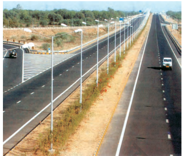
Fig. 7.2: Ahmedabad- Vadodara Expressway
